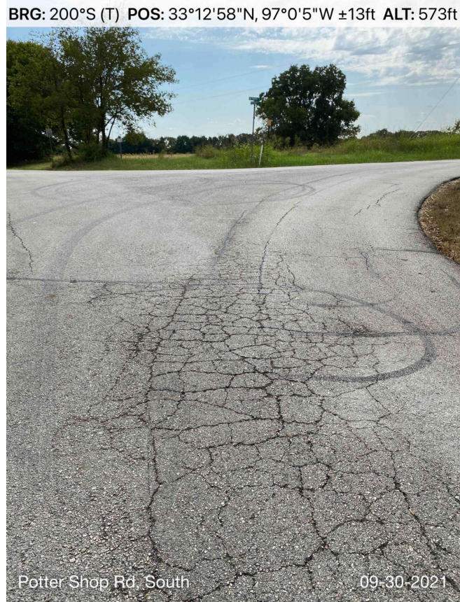
2" Mill and Overlay
