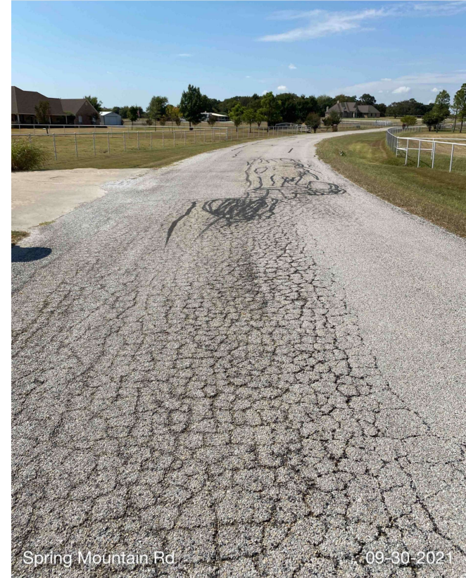
Full Depth Reconstruction
